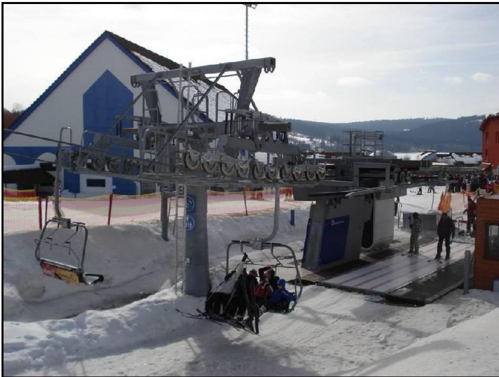
4CLF - Fixed Grip Four-Passenger Chairlift with loading carpet
